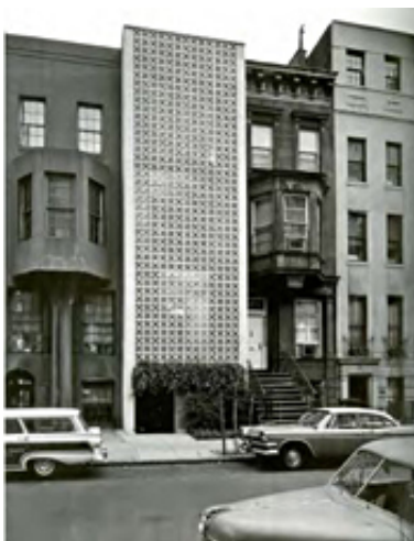
Pedro E. Guerrero Edward Durell Stone Townhouse, 1957 New York, N.Y. 1956 Edward Durell Stone, architect
