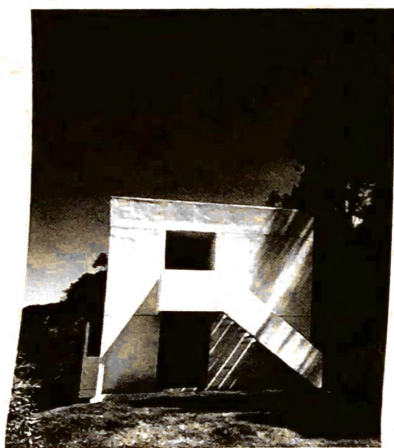
A studio addition, designed by Steven Ehrlich, was built by the second owner in 1980.
