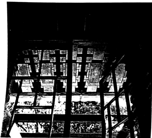
Motif painted under eaves echoes redwood trim.
